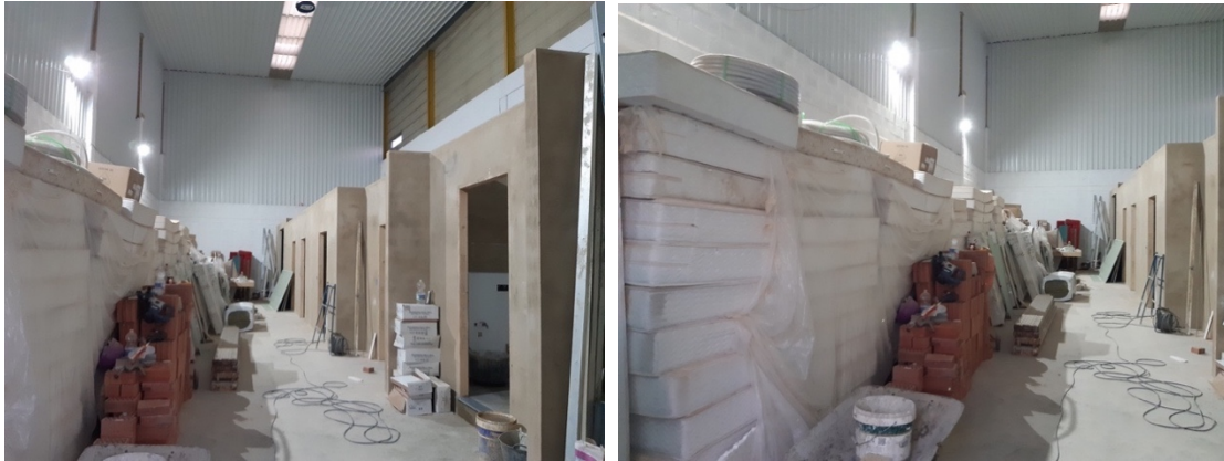
Pictures of the hostel under construction of ASNUCI in Lepe
