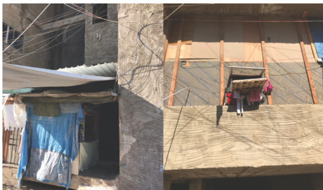
Fig. 25 Temporary closures and windows.
