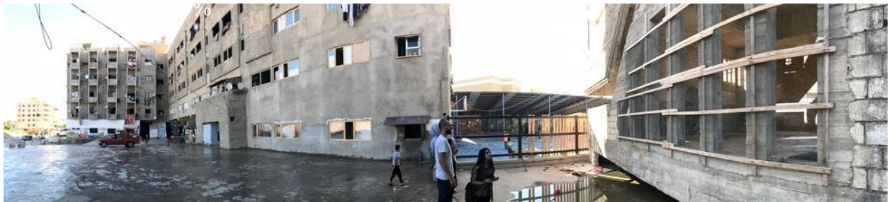
Fig. 24. Building façade of the Ouzai shelter
