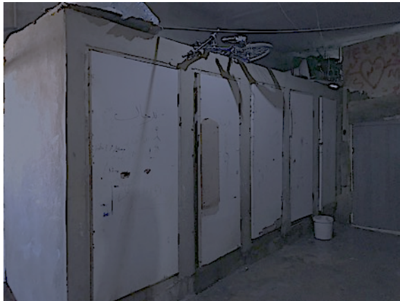
Fig. 27. Communal toilets in Ouzai shelter, Saida.
